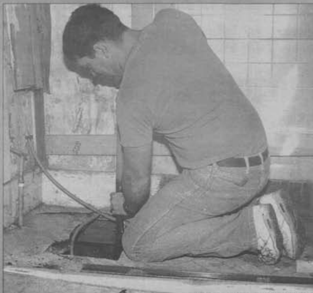
GOOD DEED - Oklahoma Army Guard's Sgt. David Gifford trenches a route for new plumbing pipes while helping to remodel the bathroom of an 85-year-old woman.
