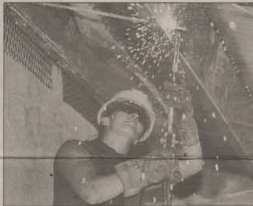
CUTTING EDGE - Spc. Bobbie Joe Williams (above) uses a cutting torch to trim roof bolts on a day care center in Ecuador.
