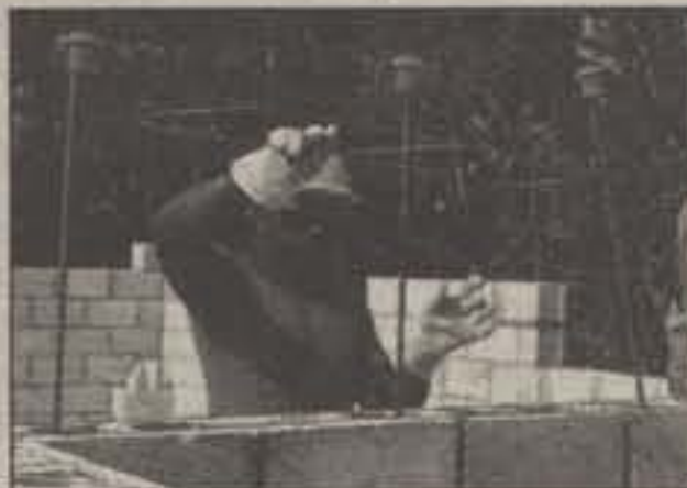
BRICK-BY-BRICK - Sgt. Herman Carraway (above) sets steel reinforcement wire while helping to build a school in Belize.
