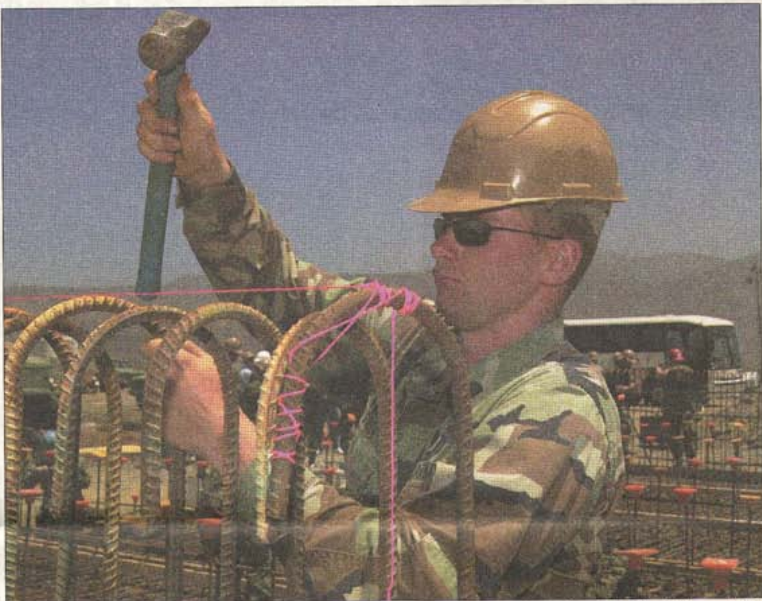
Maine Army National Guard Spc. Charlie Warren adjusts the steel rods for a concrete box culvert that citizen-soldiers from the 133rd Engineer Battalion built for the barrier system being constructed along the U.S.-Mexican border during their two weeks of annual training in southern California in May. (Below) Lieutenant Colonel David Duchring, commander of the Maine Army National Guard's 133rd Engineer Battalion, believes that "soldiers need to see their leaders in the field," even if it means climbing to the highest point on a land navigation course in the southern California desert.
