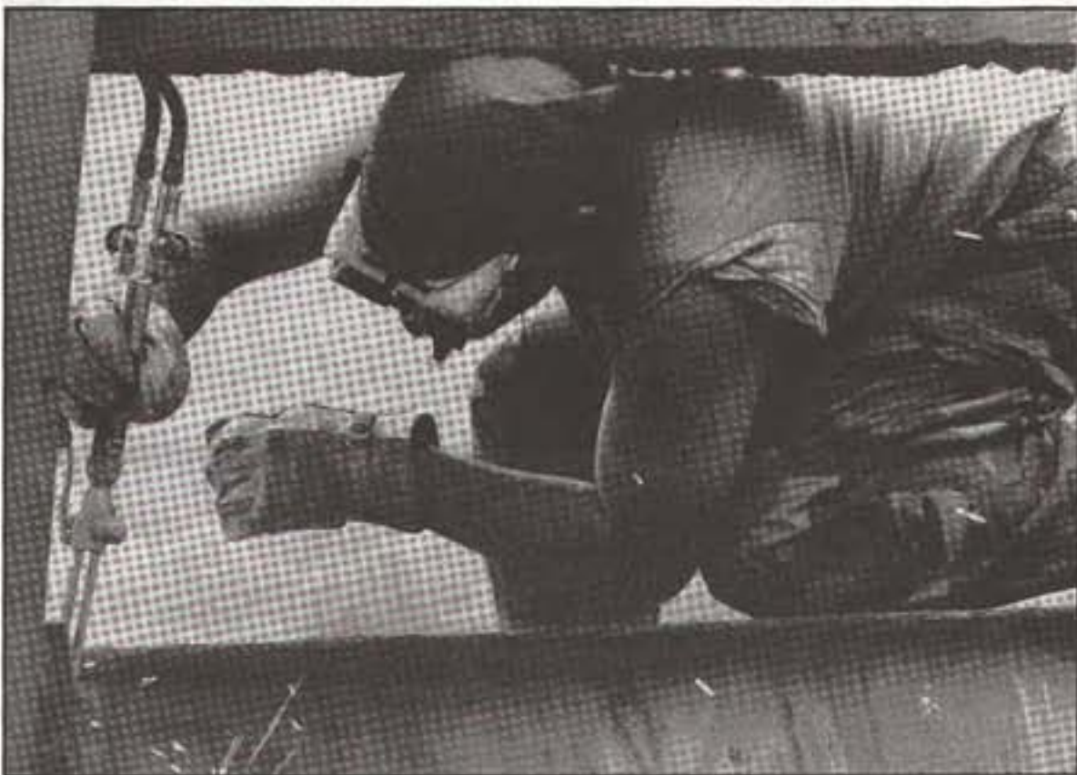
WELDING UNDERWAY - Tech. Sgt. Danny Taylor from the 124th Civil Engineering Squadron, Idaho Air National Guard cuts a steel beam from a fallen bridge in Panama. Salvaged steel was used by the Panamanians to construct other bridges. (Photo by Staff Sgt. Vern Borth, Wisconsin Army National Guard.)
