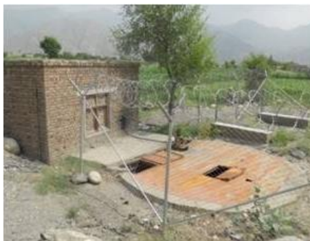
A completed solar well stands unused in Kuz Kunar. The solar panels have been removed by the villagers.
