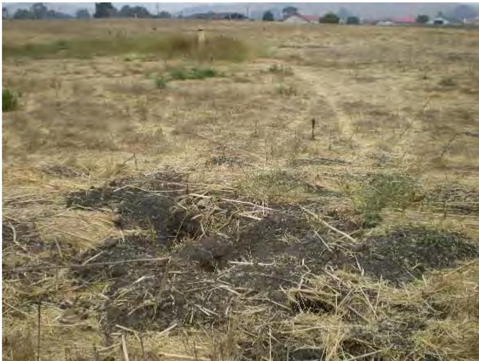
**5. Plant Growth and Windblown Debris in Grass Ditches**
