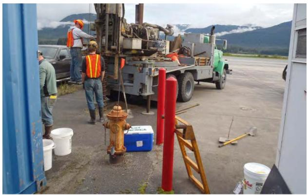
Photo 6: Drill rig advancing Boring B15. Photo taken facing south. (August 25, 2010).
