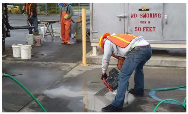
**Photo 3**: An approximately 5-inch thick block of concrete was cut from the taxiway surface to allow advancing Boring B14. This was the only boring with fuel contamination. Photo taken facing north (August 25, 2010).
