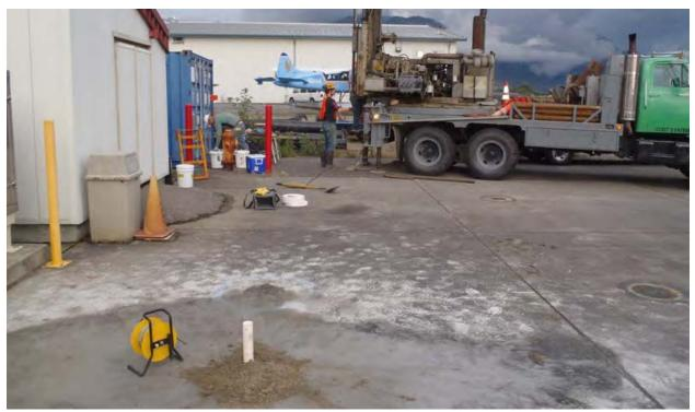
**Photo 5**: Boring B15 (being advanced by drill rig) was located near the east property boundary in an asphalt-covered area. Two-inch PVC casing for temporary well TWI is visible in foreground. Photo taken facing east (August 25, 2010).
