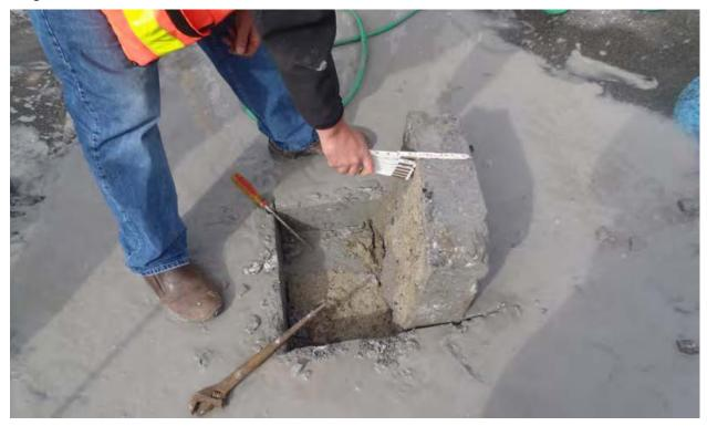
**Photo 4**: Concrete block removed at location of Boring B14 and temporary monitoring well TW1. (August 25, 2010).
