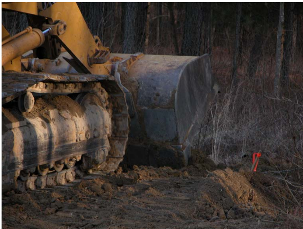
Photograph B-7. Compaction of soil with excavator bucket
