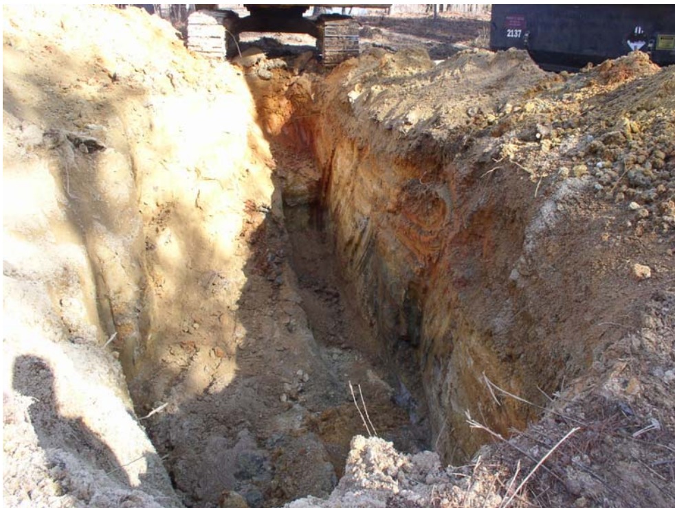
Photograph B-10. Expansion of excavation boundary to “chase” stained soils
