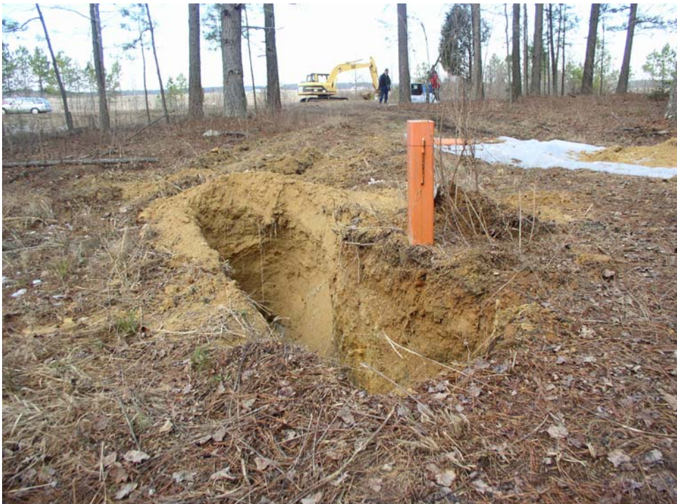
Photograph B-4. Trenching near monitoring well prior to removal
