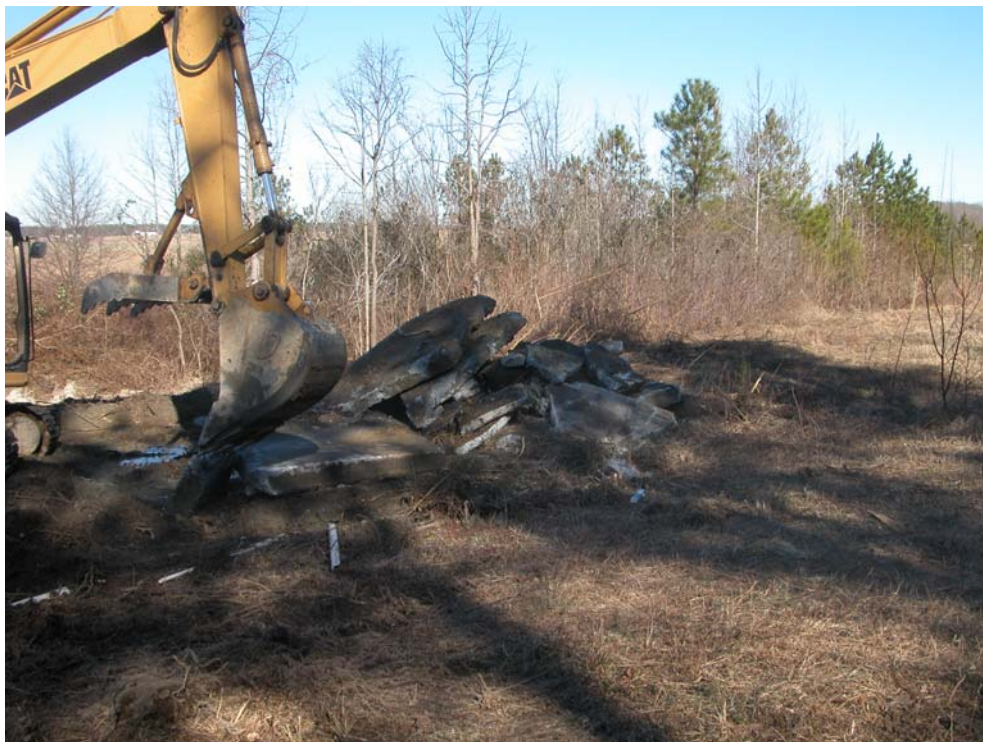
Photograph B-2. Decontamination pad removal
