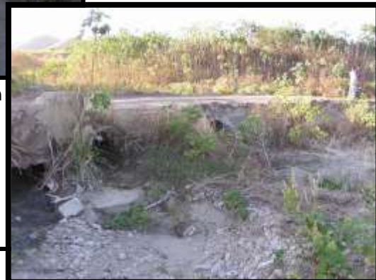
Blue Route Point 13 - Overflow
