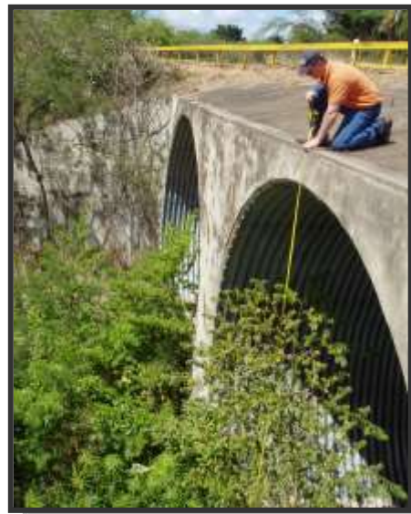
Inlet of the Quebrada Honda
