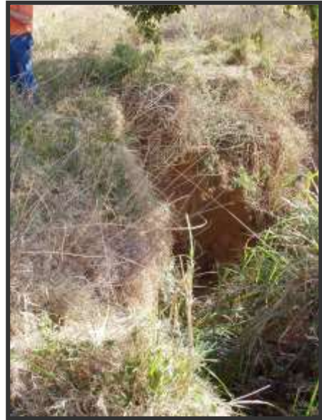
Gully along Orange Convoy Route, Point 10.
