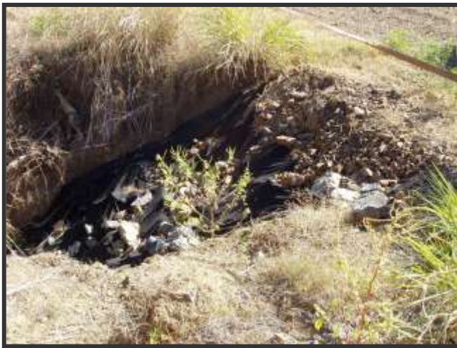
Unfinished construction along the Brown Convoy Route, Point 4
