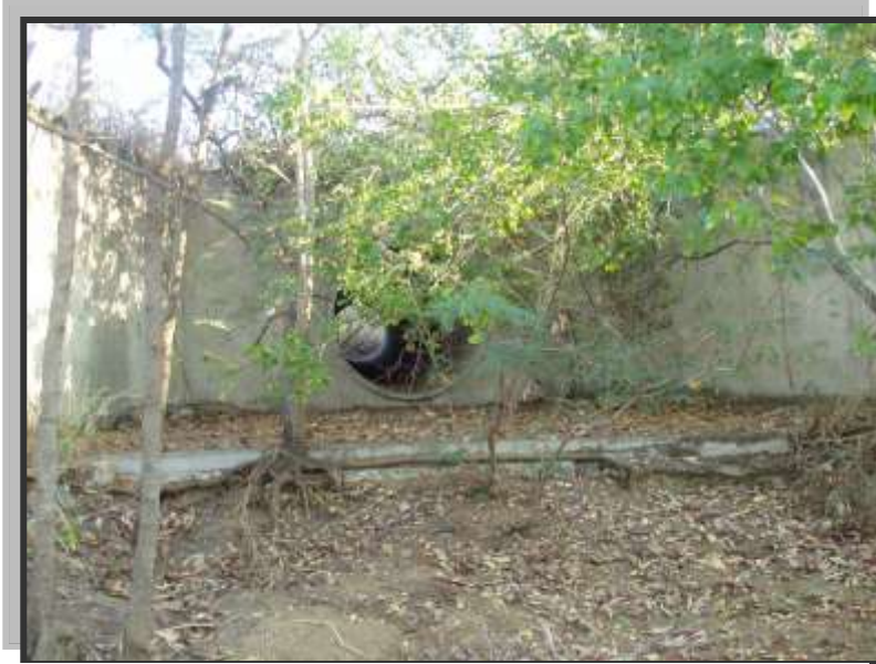
Outlet of the 60-inch crossing - Red Convoy Route Point 15.
