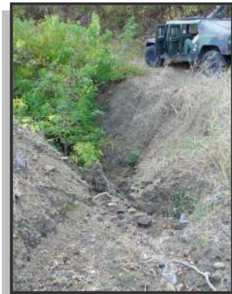
Gully along Orange Convoy Route, Point 20.
