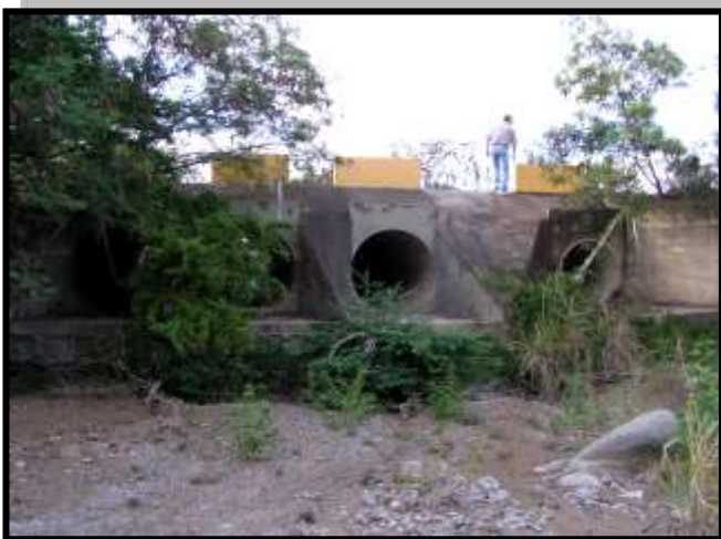
Outlet of four-barrel 60-inch crossing along Convoy Route Blue at Point 4.
