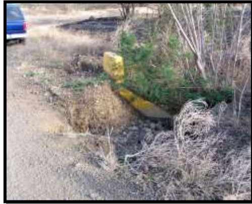
Surface drainage into stream around at crossing at Point 10 on the Blue Convoy Route.
