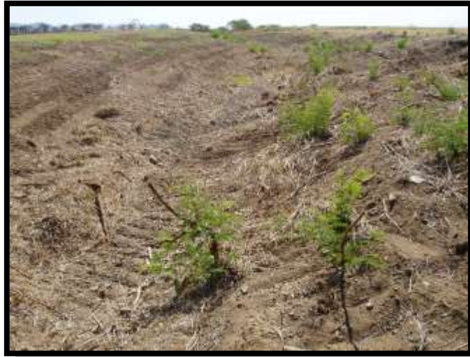
Downstream photo of channel maintenance clearing.
