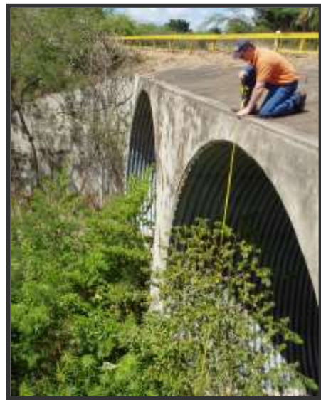
Inlet of the Quebrada Honda
