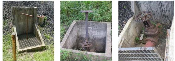
Figure 15: Various dike drain valves at CAPECO. Tank 409 fixed stem dike drain valve (left): position of the valve is undeterminable without physically turning the valve. Rising stem valves (center, right). In some cases, the valve position is hidden in the sump (center).
