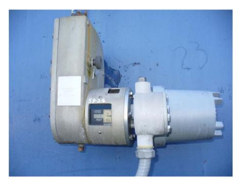
Figure 4: Side gauge: mounted on the side on a tank and displaying the amount of liquid in the tank
