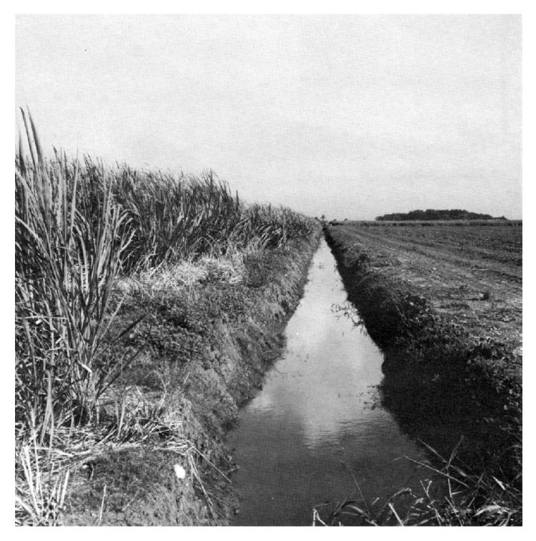
$Figure \ 3. \\ - Drainage \ ditch \ lowers \ water \ table \ and \ improves \ drainage \ of \ Coloso \ silty \ clay \ loam. \ This \ field \ is \ planted \ to \ sugarcane.$
