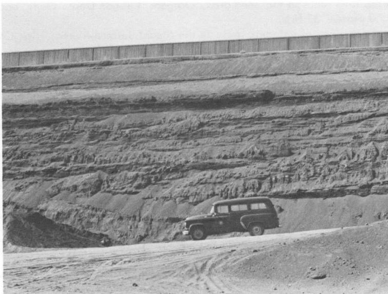
Figure 60. Knott sanitary landfill pit southeast of Bend furnishes large quantities of common fill materials used in the Bend area.
