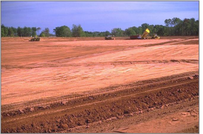
A soil cover is placed over a landfill to minimize exposure to waste and migration of contaminated surface soil via surface water runoff.
