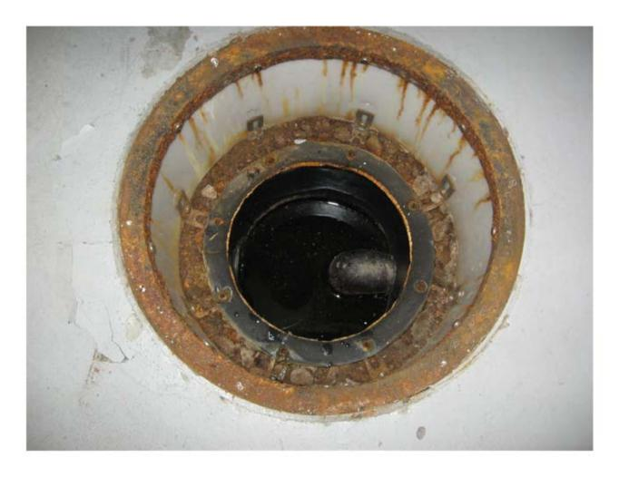
Figure 4-1. Photograph of Battery Acid Neutralization Pit in Building 636 (TU017)
