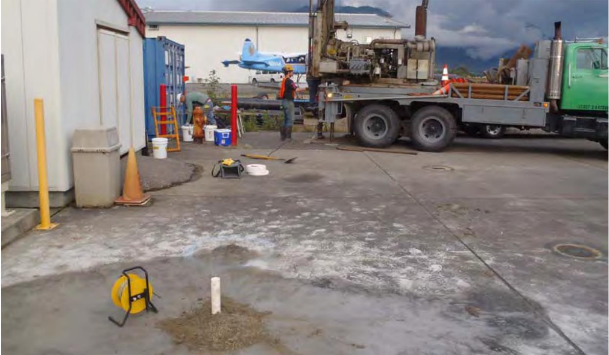
**Photo 5:** Boring B15 (being advanced by drill rig) was located near the east property boundary in an asphalt-covered area. Two-inch PVC casing for temporary well TWI is visible in foreground. Photo taken facing east (August 25, 2010).
