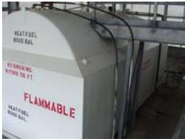
Stop flow of spill by closing valves, uprighting container, or creating a berm with boom, dirt or snow. Piping shut-off valves are placed at several locations in the fuel piping network.
