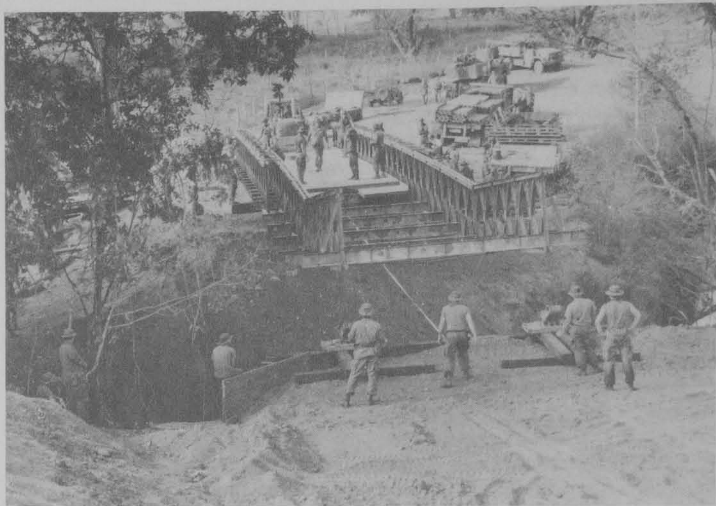
ARNG engineers emplace a bridge in Panama.
