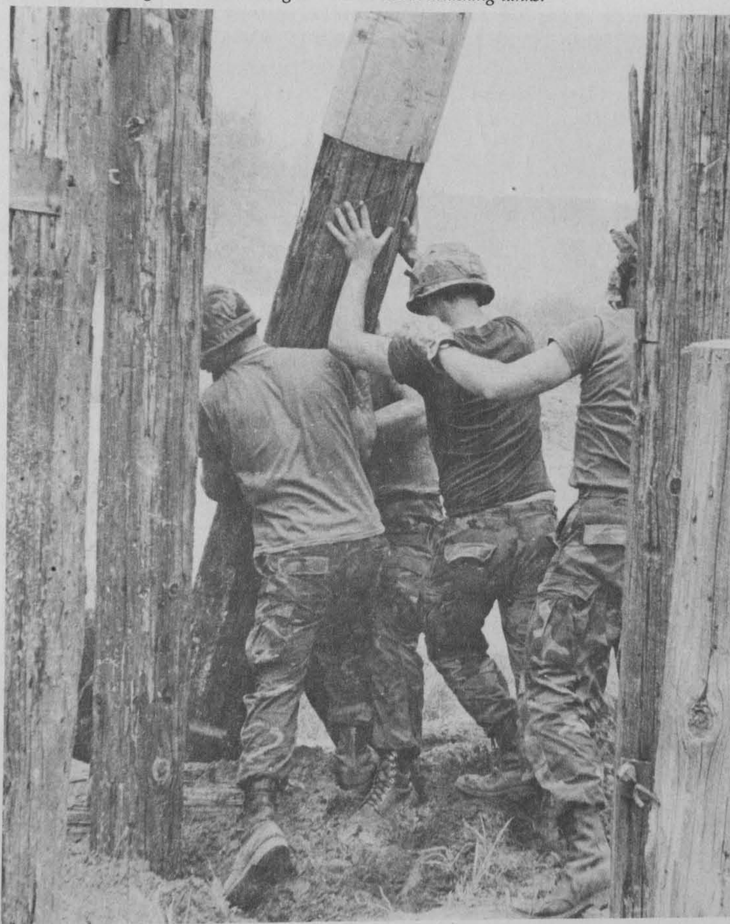
Soldiers from Company D, 724th Engineer Battalion, Wisconsin ARNG, erect a log crib obstacle designed to slow down attacking tanks.
