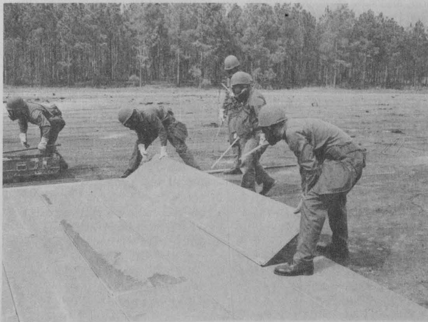
In field gear and protective masks, members of the 142d Civil Engineering Flight, Oregon Air National Guard, repair simulated runway bomb damage with metal mats during AT at Eglin AFB, Fla.
