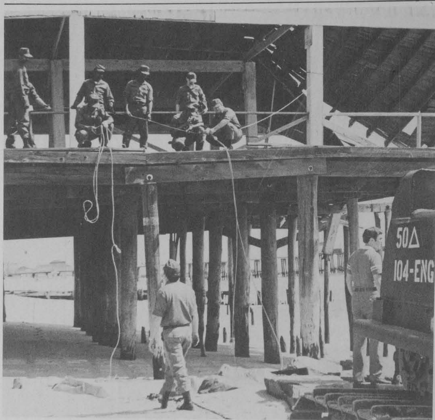
The fierce winter really hurt the shore. To help get it back into shape, members of the 104th Engineer Battalion tore down a heavily damaged pavilion and bulldozed sand back into place in Ocean Grove.
