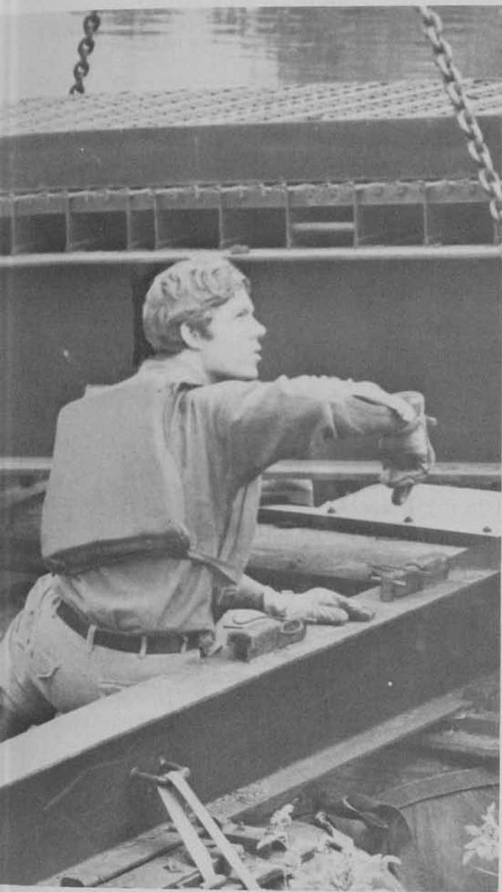
Oregon Army National Guardsman bolts sections of a floating bridge in place during Annual Training at Camp Rilea, Oregon.
