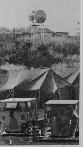
Maintenance tents support the operations of the Air National Guard AN/TRC-97 Tropospheric Radio System in the foreground and the Radar Operations Center on the right during Spring 1974 field exercises.
