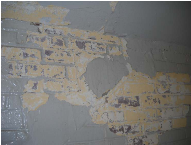
Room D-9T-S (men's restroom), peeling blue paint
