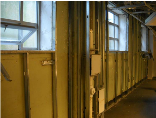
Room 12-W ("Microbial Hazard"), wall studs following drywall removal
